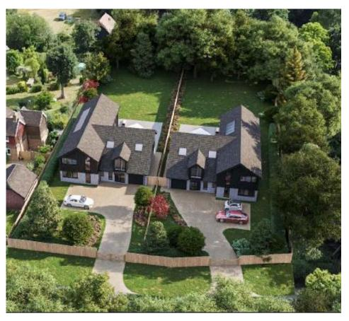
2.02 The houses have a mix of gabled and catslide roof forms with slate effect roof tiles, external walls would be finished with a 'light facing brick' at ground floor level and grey vertical cladding at first floor. Windows are doors would be grey aluminium.
